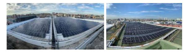
The total generating capacity of solar panels at Serangoon North Cluster and K&S Corporate Headquarters is 848.8 kWp.
